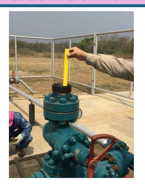
THE REMOVAL OF A PERCENTAGE OF THE WATER COLUMN ALLOWS THE WEIGHT OF THE REMAINING WATER TO FALL LOWER THAN THE STATIC PRESSURE BARRIER, WHICH CAUSES THE WELL TO DISCHARGE ITSELF.
